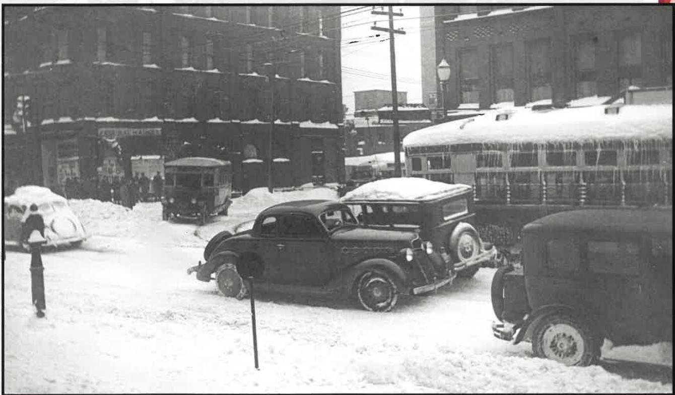
Getting around town in a Western New York winter can be a challenge, whether driving or using public transportation, as this St. Patrick's Day view of the intersection at West Third and Washington streets in Jamestown demonstrates. Check out the icicles on the rail car windows in this 1936 photo! COURTESY FENTON HISTORY CENTER
