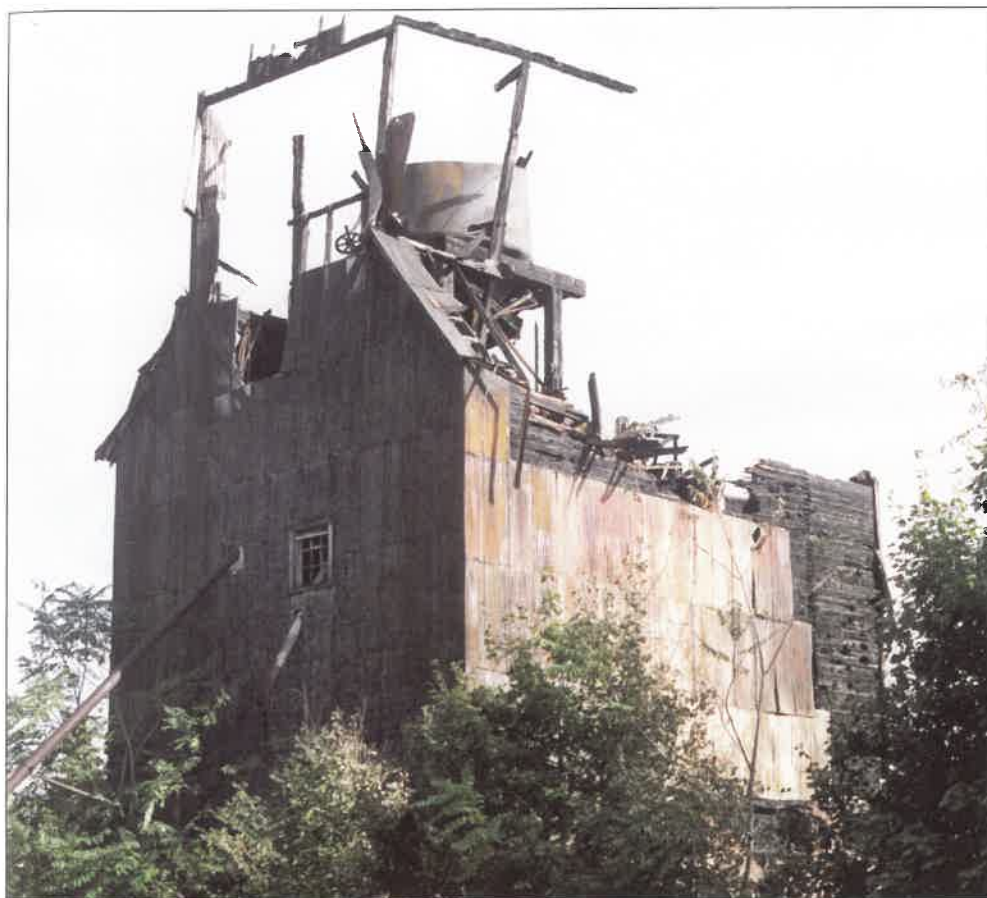
Ruins of the Wollenberg Elevator, view from the northwest JOHN H. CONLIN PHOTO, OCTOBER 2006
