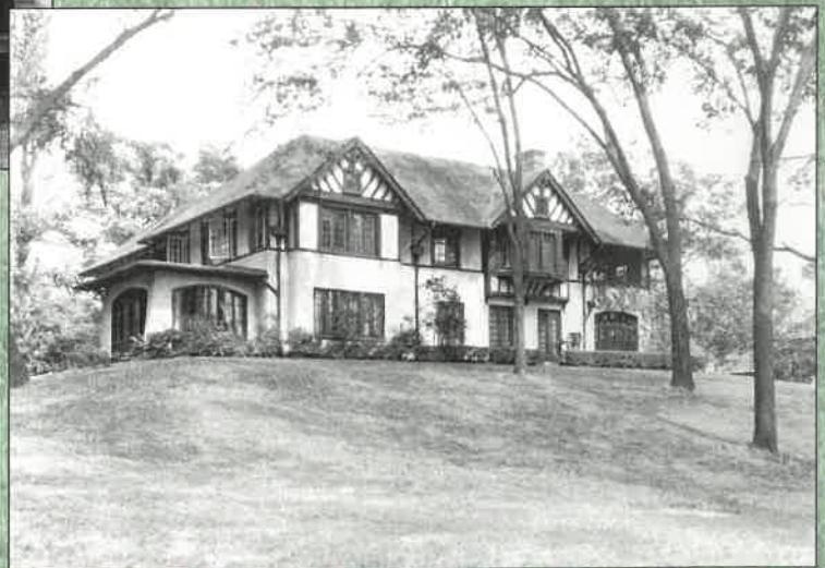
Charlotte died in 1934. New York State acquired Riverlawn in 1935 to become part of Beaver Island State Park. All of the houses were demolished for the development of the park in 1935 except the Tudor Revival house shown here. Built in 1911, and designed by the firm of Lansing, Bley & Lyman, it was the summer home of Charlotte's son Ralph Sidway.
