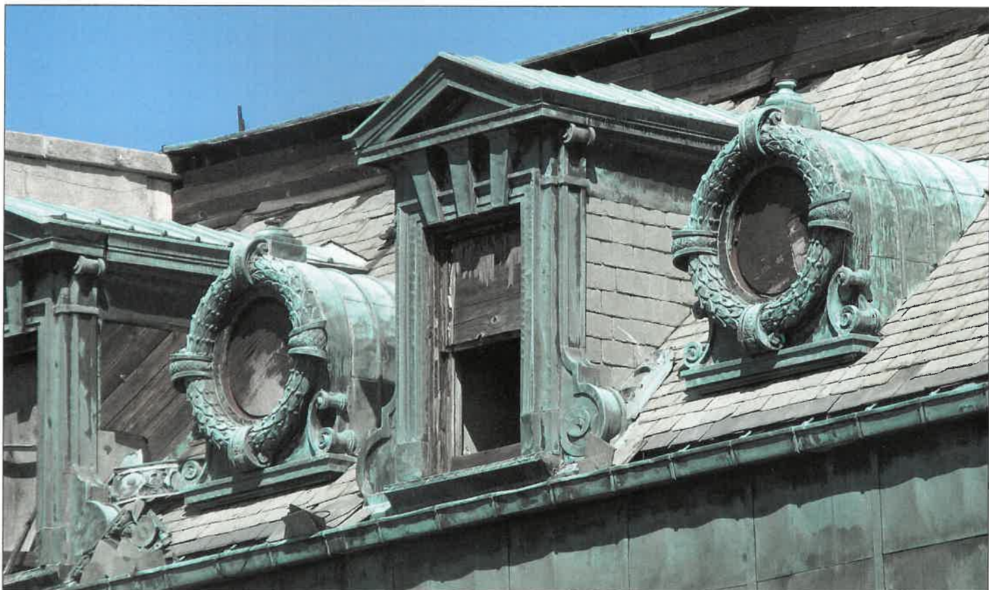
Detail of the southern roof elevation, showing the elaborate copper dormer décor—as well as evidence of the building's decline. DOUGLAS W. DeCROIX PHOTO, 2009
