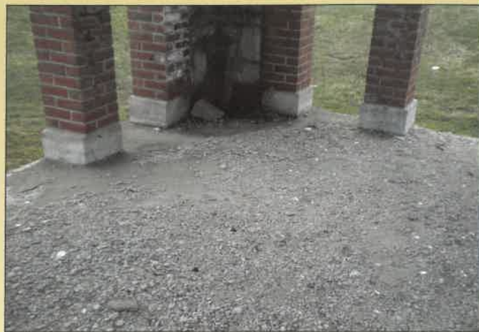
Though the cement foundation shows decay, preservationists believe it could still be moved if that were determined to be the best course of action. PHOTO BY DEAN GOWEN
