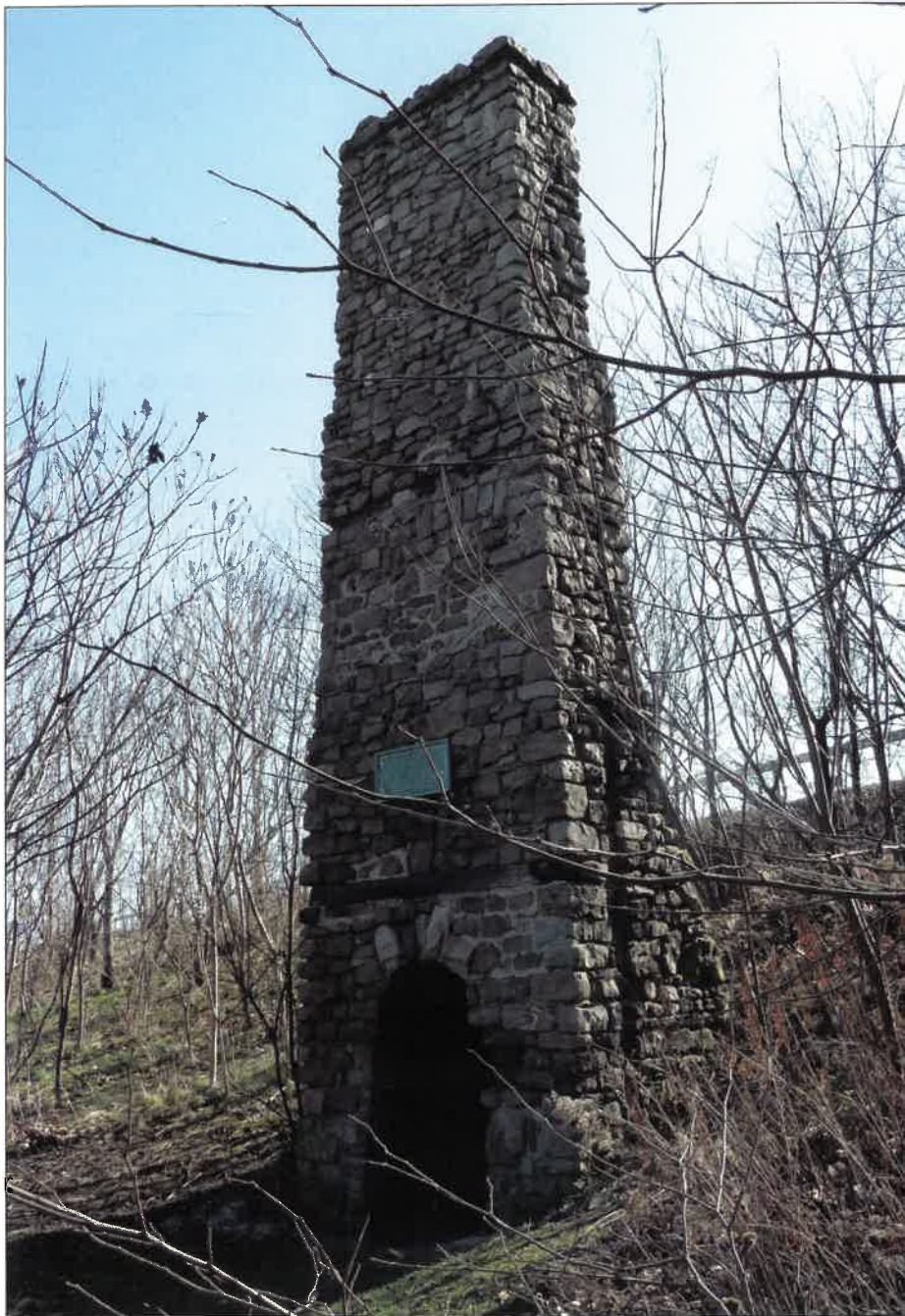
Today, the chimney is nestled against the embankment of an off-ramp to the Robert Moses Parkway, but plans to reconfigure the parkway once again place this irreplaceable artifact at risk. CHRIS PUCHALSKI PHOTOGRAPH, 2013
